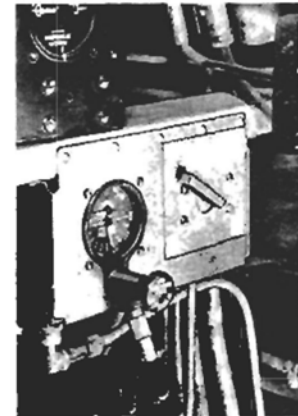
Figure 11—Pilot's Oxygen Regulator
